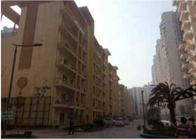
Low Rise Towers
